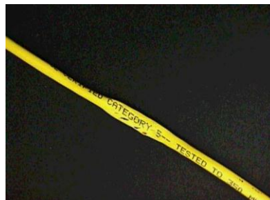
Photo 11: A cable that has been smashed or crushed. Note the cuts in the outer cable jacket
