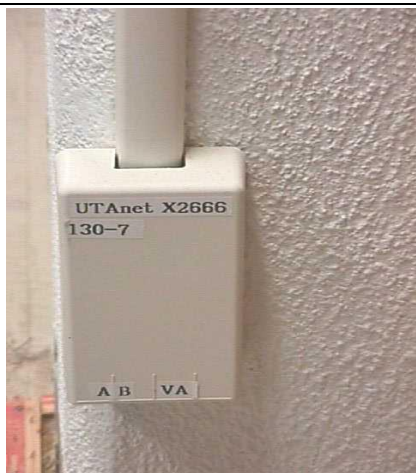
Photo 18: Example of 4-port PANDUIT surface mount box (P/N CBX4IW-AY).
