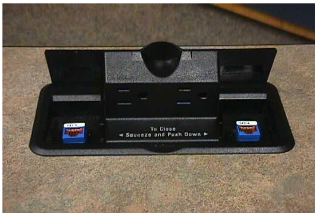
Photo 27: KI PowerUp Module with Panduit Keystone jacks installed.
