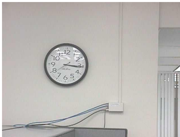
Photo 21: Example of exposed raceway application. Mounted on a non-hollow wall above the level of the modular furniture.
