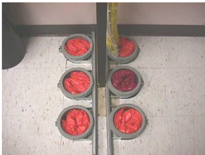
Photo 32: Properly Fire-stopped using SpecSeal™ Intumescent Pillows
