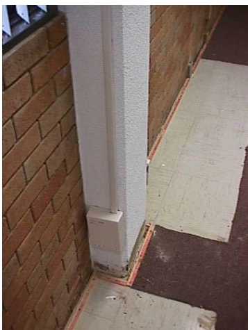
Photo 20: Example of exposed raceway application. Attached to the pillar.
