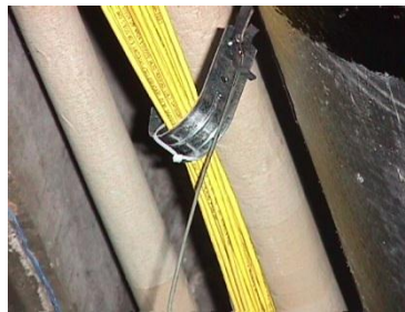
Photo 12: Proper use of CADDY J-Hooks.
