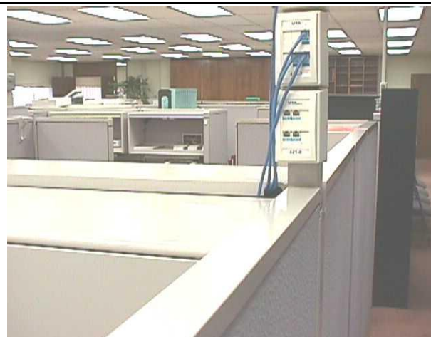
Photo 19: Example of one-piece single gang junction box (P/N JB1IW-A) mounted to a power pole to feed the top caps of modular furniture. Junction boxes are faced with PANDUIT Brand Executive style Mini-Com faceplate (P/N CFPE6IWY).
