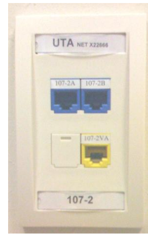
Photo 23: Picture of Proper Faceplate Configuration
