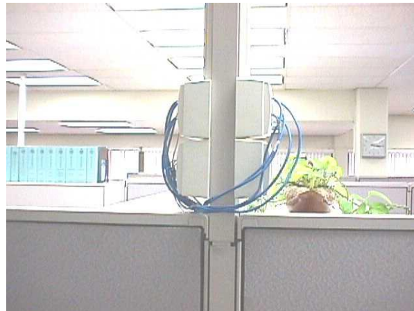
Photo 24: Example of single gang surface mount boxes with executive faceplates mounted on a power pole feeding top-caps.
