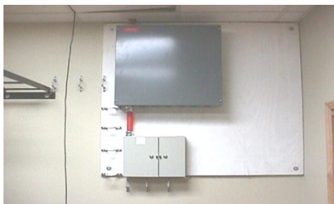
Photo 29: Wall Mount Enclosure and Fiber Slack Enclosure.
