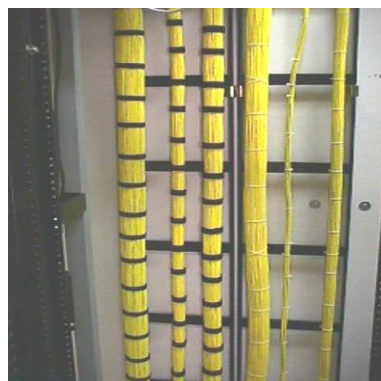
Photo 7. Proper transition between floors. Bundles are correctly secured to vertical ladder sections by cable ties or Velcro straps.
